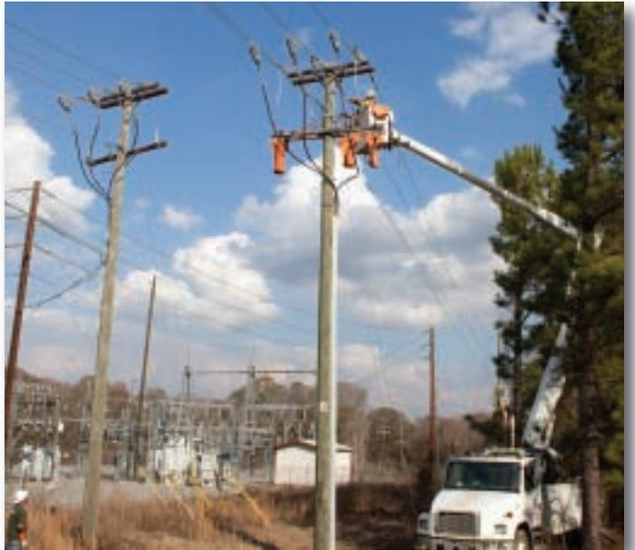
▲ Contractors restructure lines outside of the Walkerville Substation to prepare for the new circuit and conductors.
